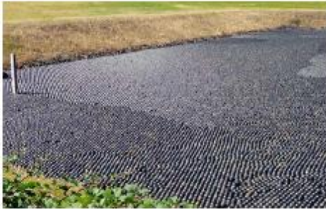
Bird balls keep canadas and other waterfowl out of retention ponds
